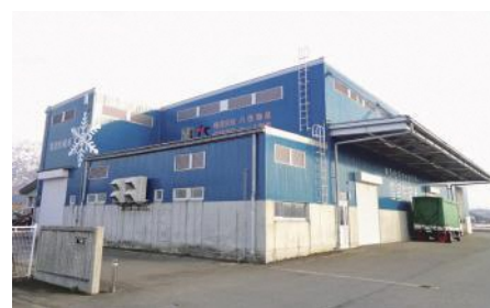
06 [米穀] 八色物産雪室貯蔵庫
